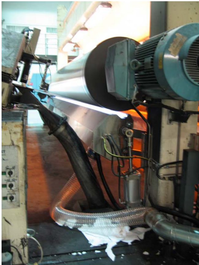
Inspection beam (below the roll) and its pneumatics cylinder as well as low pressure (cooling) air pipes seen from the drive side.
